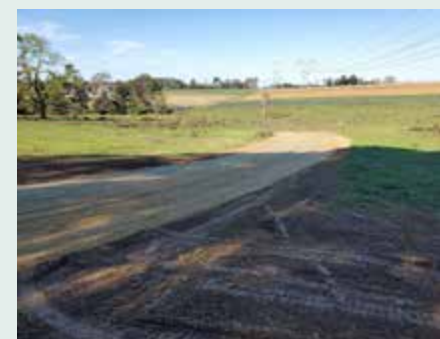
Waterway after matting.
