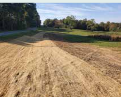
Diversion after matting.
