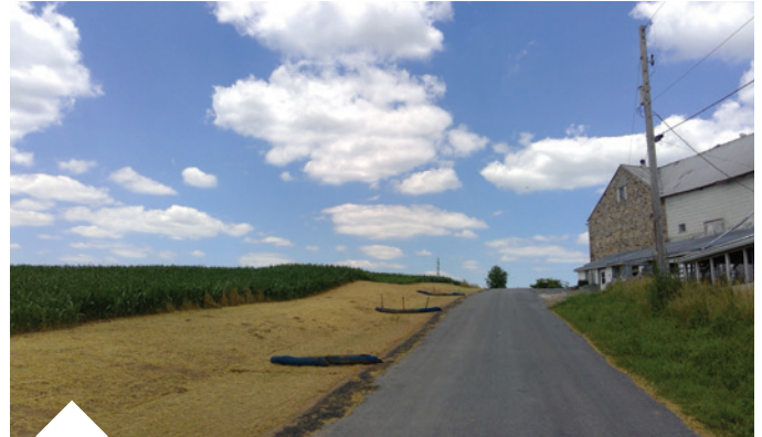
Swale development to control stormwater on Twin Hill Road
