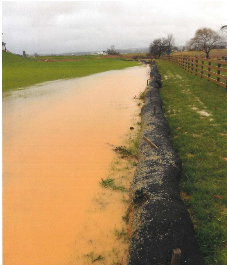
A compost filter sock working and keeping sediment-laden runoff on-site. Photo by Alex Flurry - LCCD
