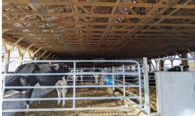
A roofed heavy use area.
