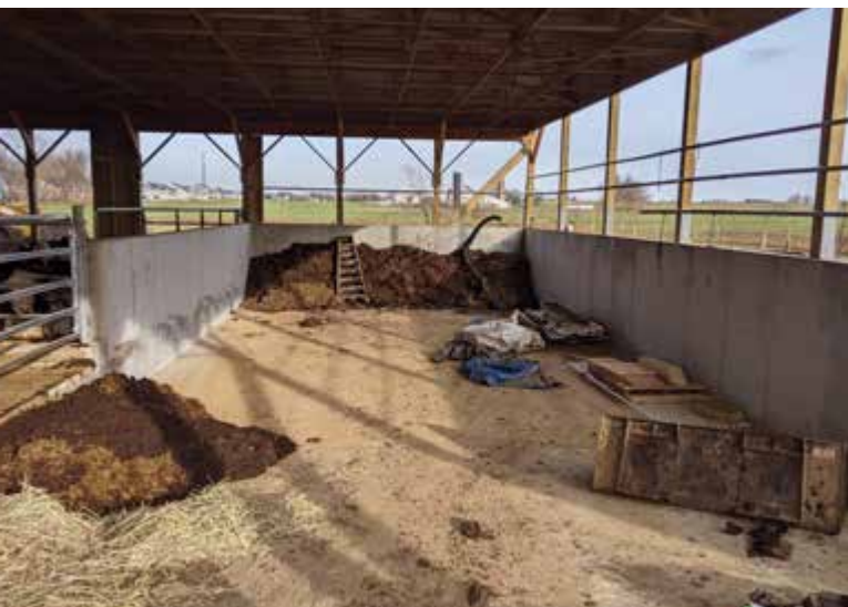
A roofed stacking area for manure.
