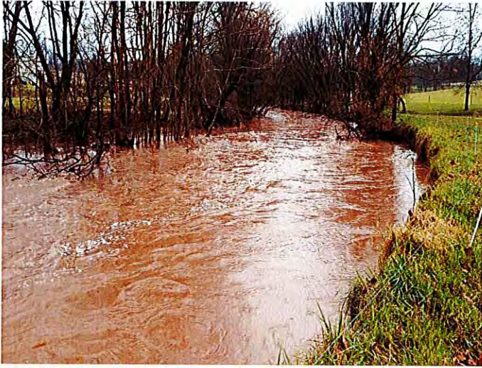
Site photos showing problems to be addressed
