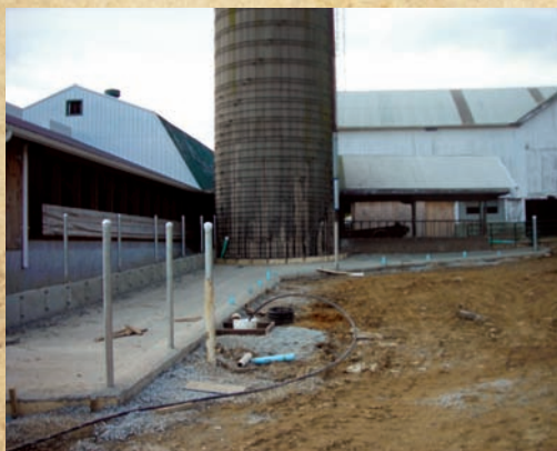
A barnyard under construction to collect runoff and direct it using conservation practices.
