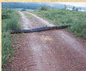
Conveyor Belt Diversion installed on a Dirt & Gravel Road.
